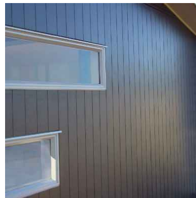
CFC CLADDING EXPRESSED JOINT
