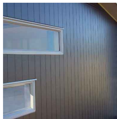
CFC CLADDING EXPRESSED JOINT
