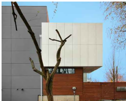
CFC CLADDING EXPRESSED JOINT
